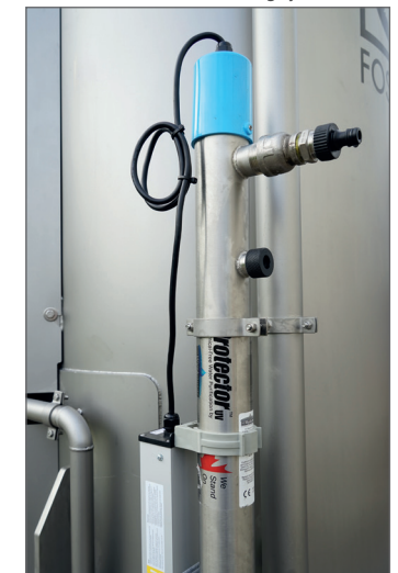
Water disinfecting system on ICU
